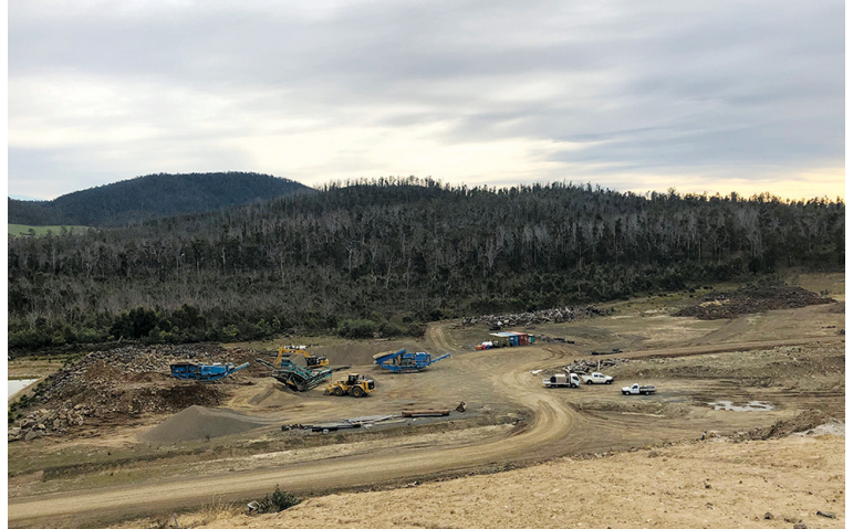
Looking out from the top of the landfill at what will become Stage 2
